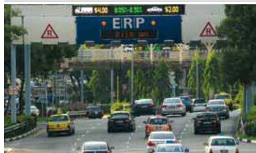
Figure 2: ERP gantry with real-time display of ERP charges
